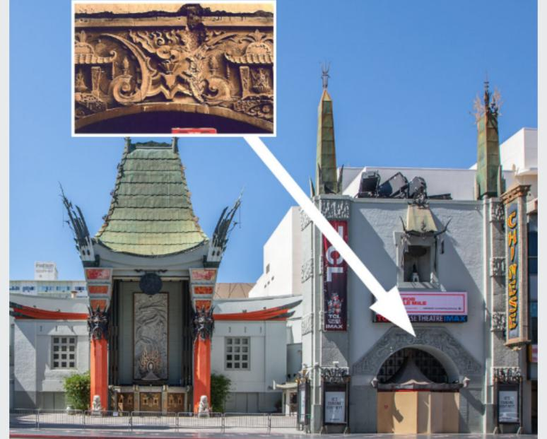
This photo shows one of the cast stone architraves and its location within the overall building façade. The architrave was covered-up in 1958 with a neon sign. Inset picture shows damage to architrave prior to restoration (© Amy Higgins)
