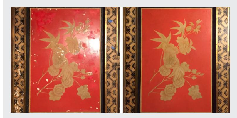
Closeup of lobby ceiling panel showing "before" and "after": water-damaged surfaces (left) and subsequently repaired surfaces (right) Image © Amy Higgins
